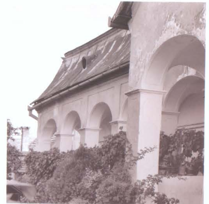
5. The spacious porch is an inalienable part of the Armenian house; its prototype is the loggia of Renaissance palaces
